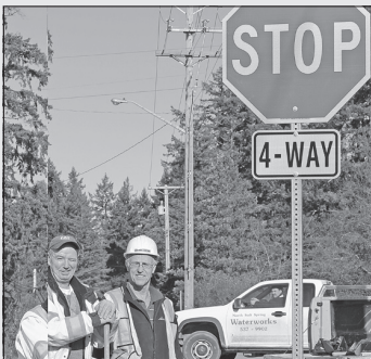
Brian Pickford and Dale Johnson of Mainroad Contracting with four-way signage at Central.
