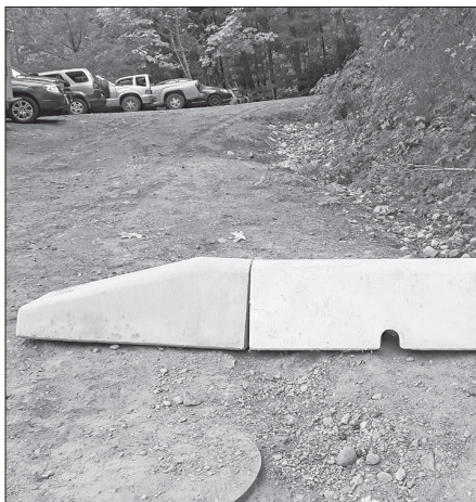
Barrier placed near Burgoyne Bay dock to help reduce erosion of the road. PHOTO COURTESY HASSI
