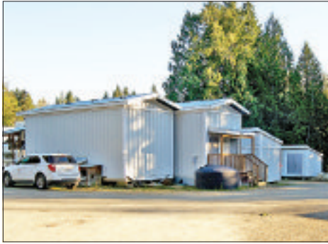
The abattoir facility on rented land a few kilometres south-west of Ganges.
