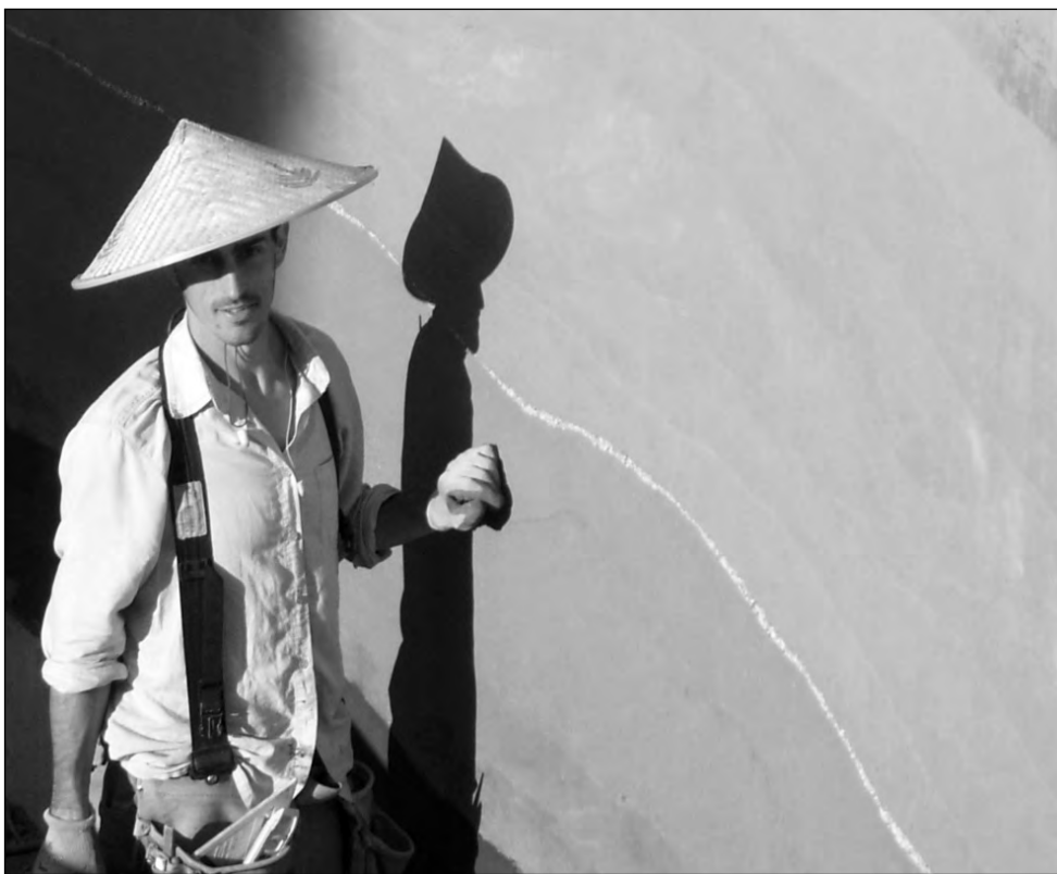
Clifton Schooley completes work on the West Coast's largest rammed earth walls on the grounds of the University of British Columbia's botanical gardens.
