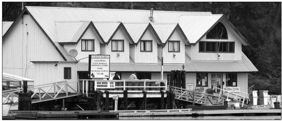
A seaside view of the floating structure at Ganges Marina.
