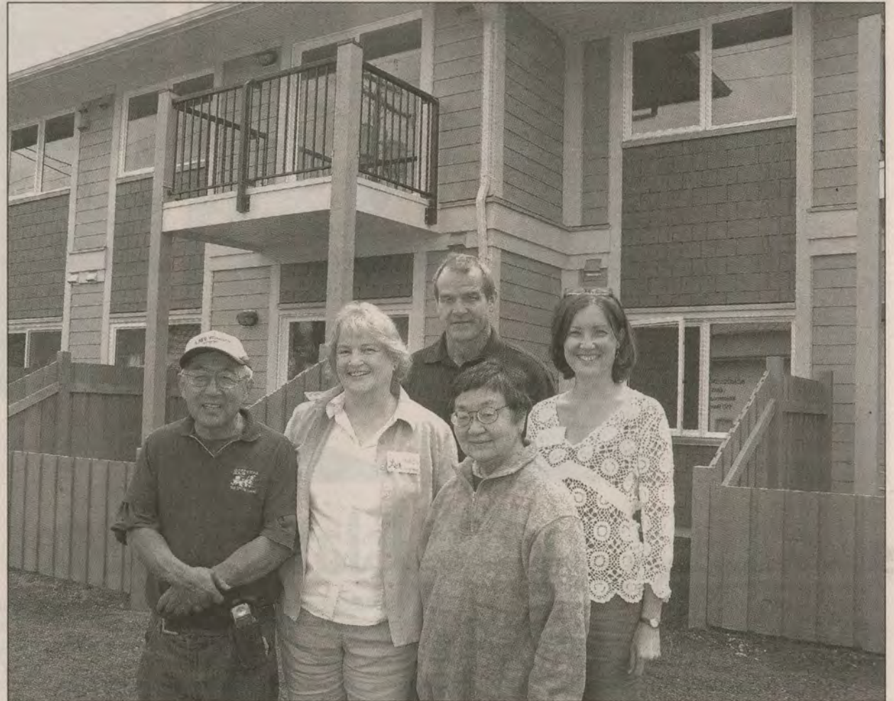
Affordable housing complex Murakami Gardens opened its doors to its first tenants in 2008.
