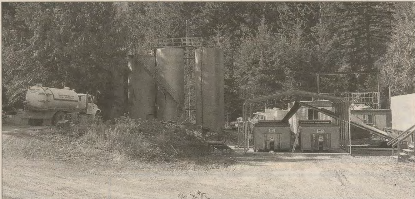
Existing facilities at the CRD's Burgoyne Bay liquid waste site are deemed in need of capital upgrades.
