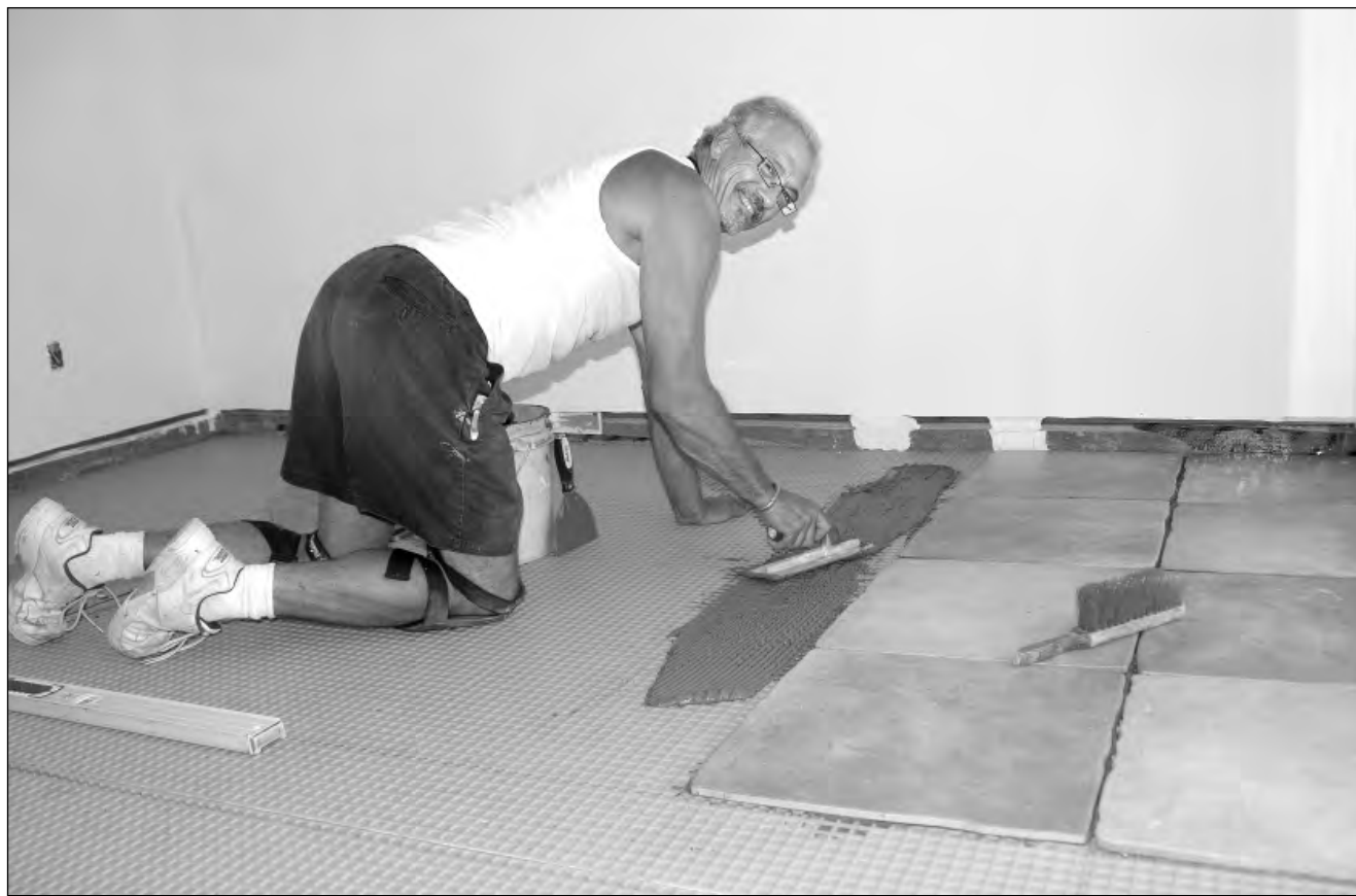
TOUCH OF TILE: Don Monteith works on tile installation at a house on Salt Spring.
