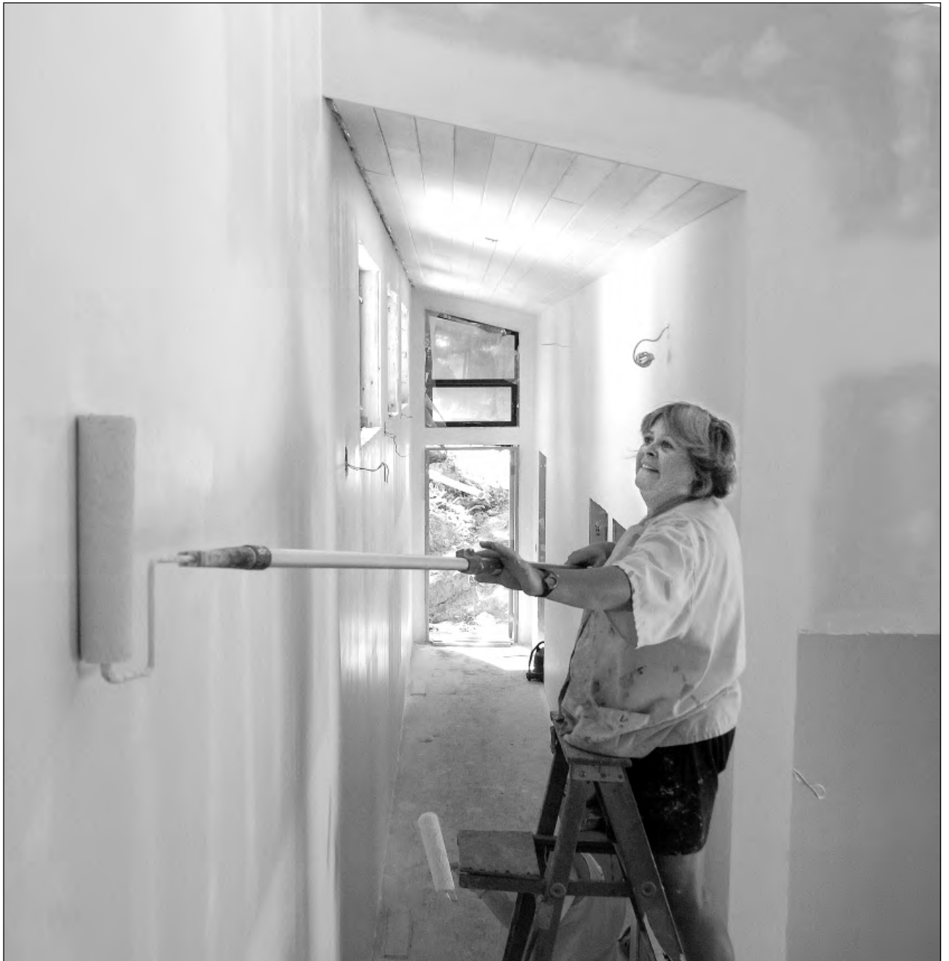
FRESH LOOK: Deb Stevenson paints a freshly dry-walled house under construction on Salt Spring.
