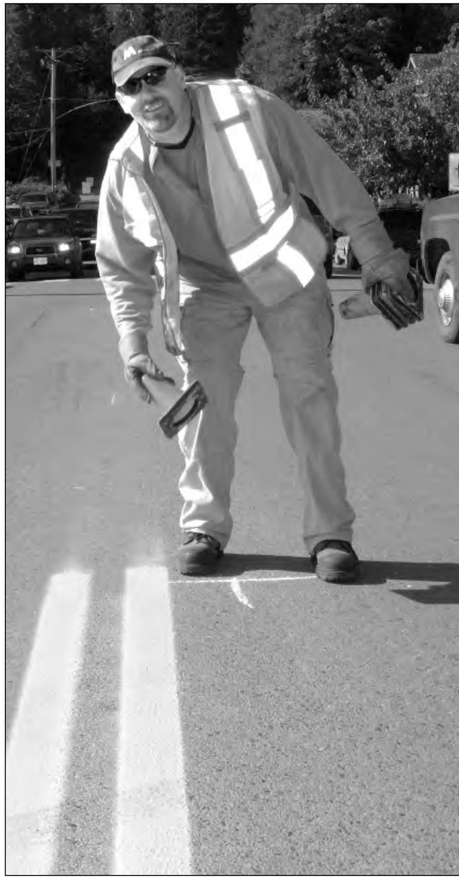
NEW LINES: Mike Pighin, of Mainroad Contracting, works on line painting as Salt Spring roads get a touch-up.
