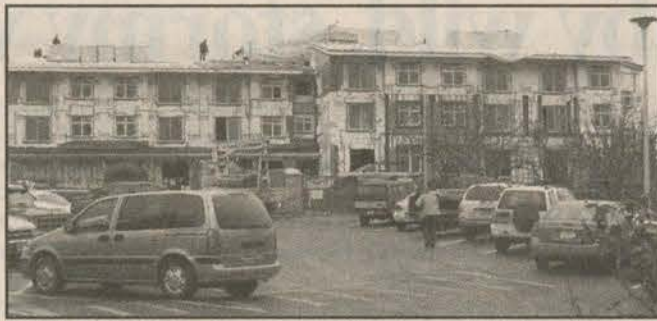
ON THE RISE: Greenwoods' assisted living facility construction is on track.
