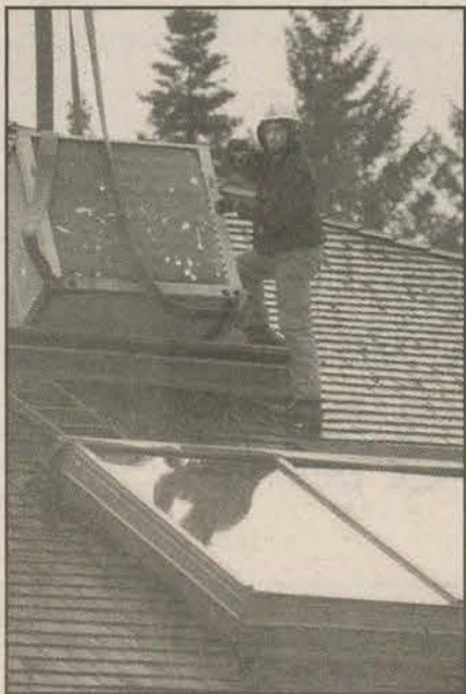
OUT WITH THE OLD: ArtSpring roof ventilation system is removed.
