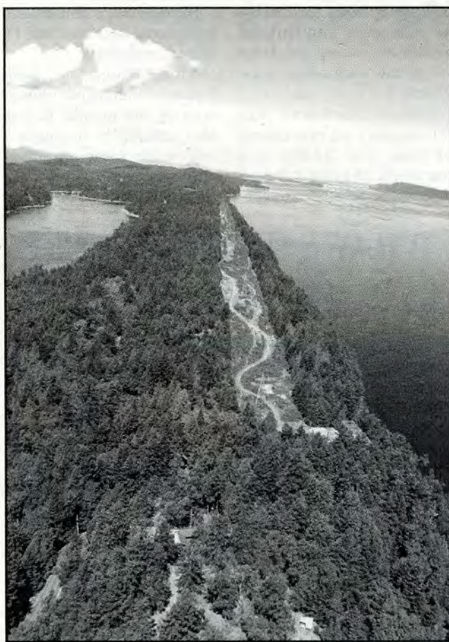
BIRD'S EYE VIEW: Power lines in Salt Spring's Long Harbour area as seen from the air. Photo by Peter McCully
