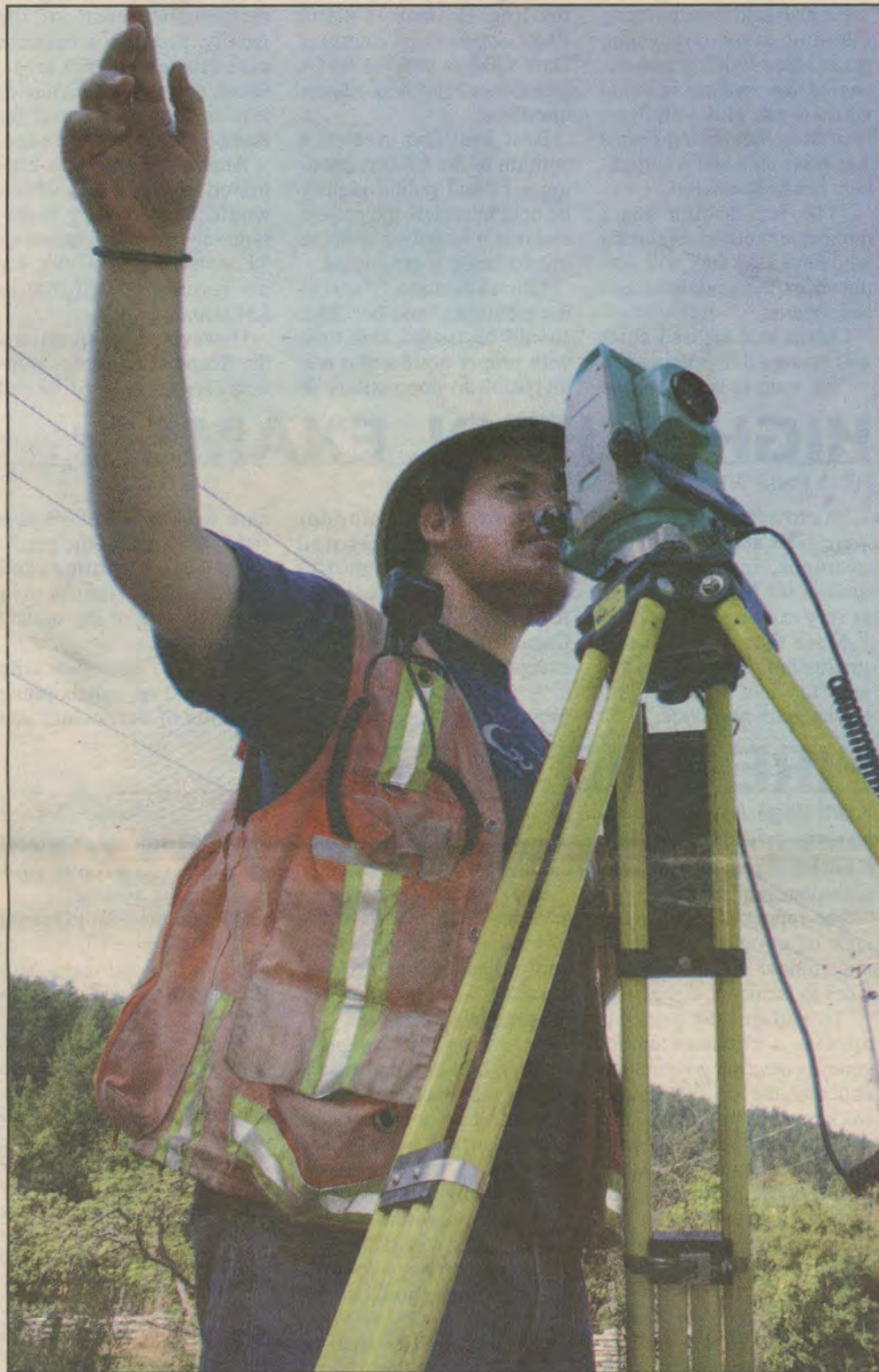
SURVEY SAVVY: Derek Adams with Bullock-Baur Associates surveys the initial layout for a retention pond at the forthcoming recreation centre on Rainbow Road. Photo by Derrick Lundy
