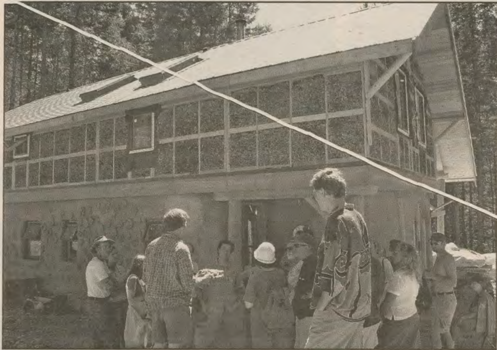
HOUSING EVOLUTION: Participants learn how discarded blue jean clippings help insulate residents in this cob home located near Bader's Beach. The home was on Sunday's Eco-Home Tour, which attracted more than 400 people. Photo by Sean McIntyre
