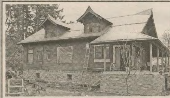
Booth Bay Restoration in Progress Available soon for your project
