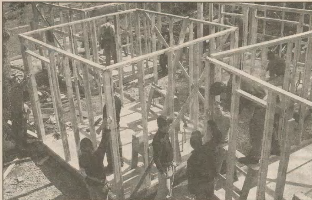
FRAMED: Students in the carpentry program at Gulf Islands Secondary School learn the ins and outs of framing small structures. Photo by Derrick Lundy
