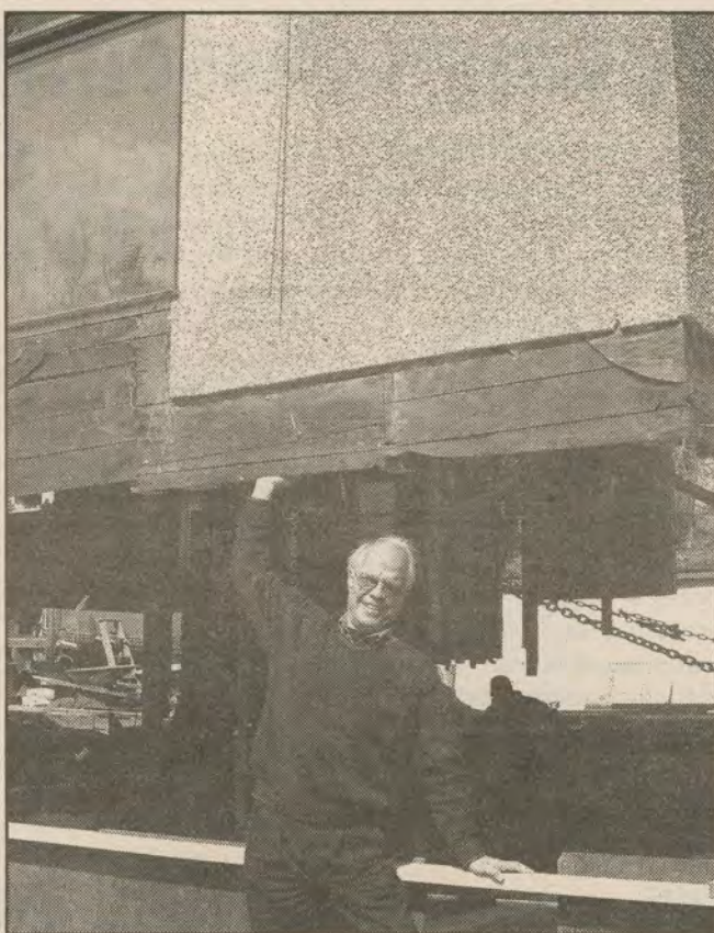
GANGES RENO: Jeremy Milsom "holds up" the "cactus" building on Hereford Avenue as the structure undergoes a renovation.
