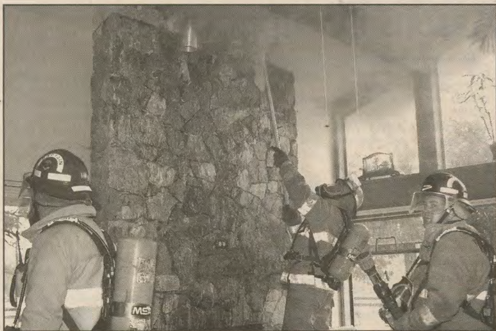
FIGHTING FIRE: What began as a routine chimney fire on the morning of Wednesday, March 9 turned into a full-fledged structure fire that forced fire-fighters to spend much of the day dismantling the chimney of an older home on Scott Point Drive. Photo by Derrick Lundy
