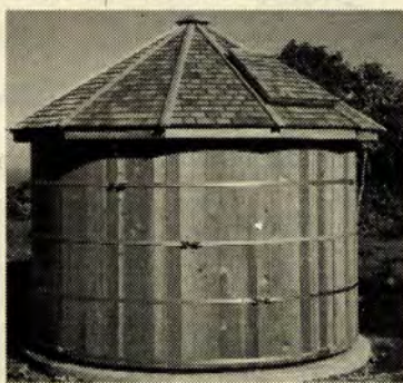
6500 gal., 8ft high sides and 12ft in diameter
