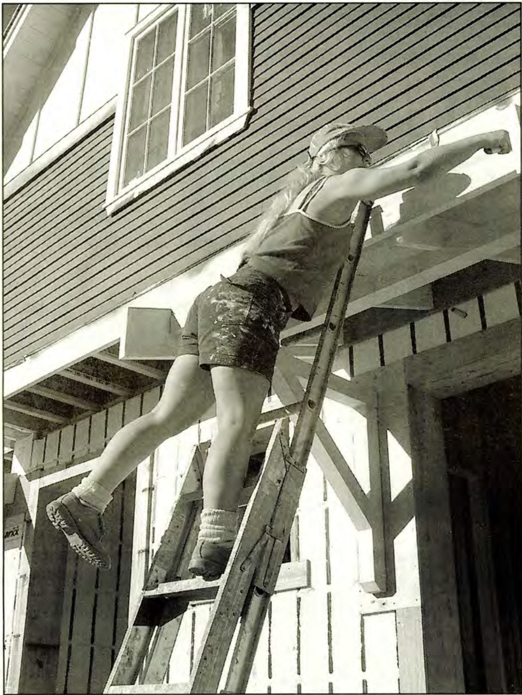
KERRY TRUSSLER , who recently moved to Salt Spring Island, stretches to put the finishing touches on one of the townhomes at Summerside. 9:30 a.m.
