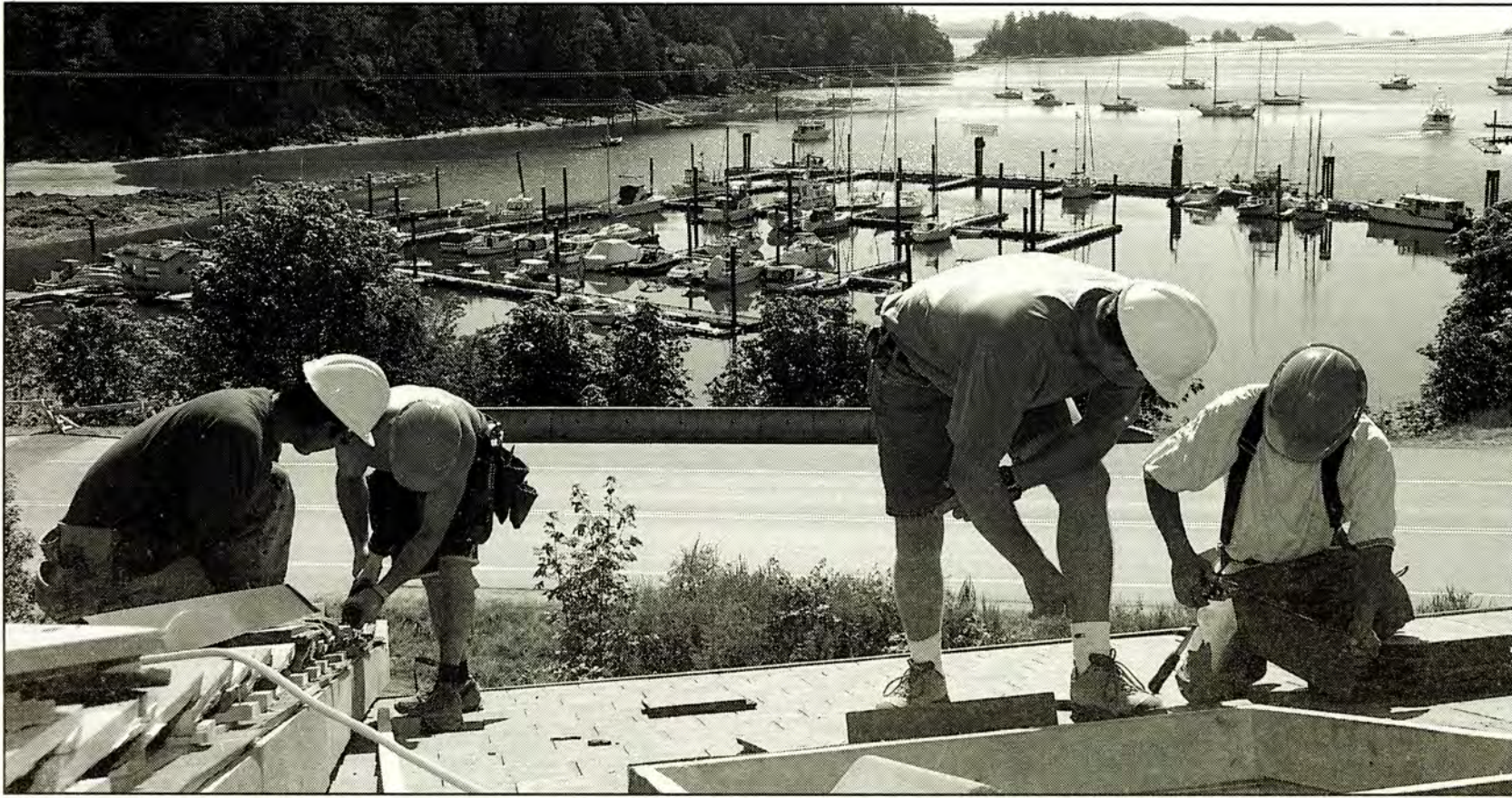
IAN WILSON instructs Martin Hooper, Jeremy Smith and Leon Lafortune how to lay the cement tiles around a skylight at a construction site at the mouth of Ganges Harbour. 2:00 p.m. photo by Derrick Lundy
