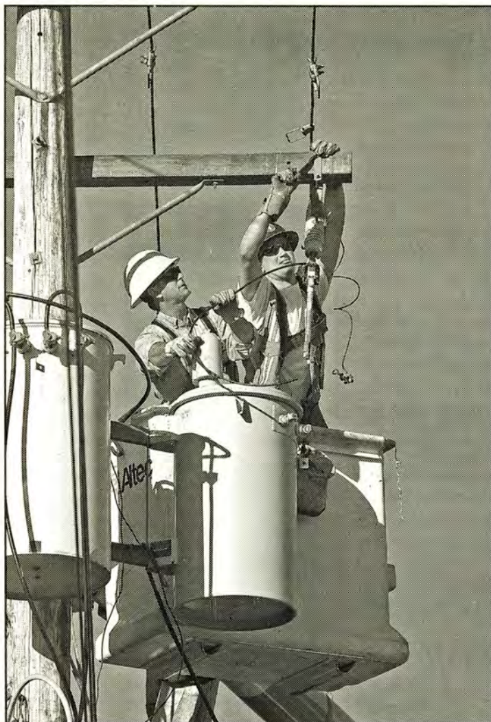
RICK BISSETT and Kirk Kid install a new transformer in downtown Ganges at 6:30 a.m. photo by John Cameron
