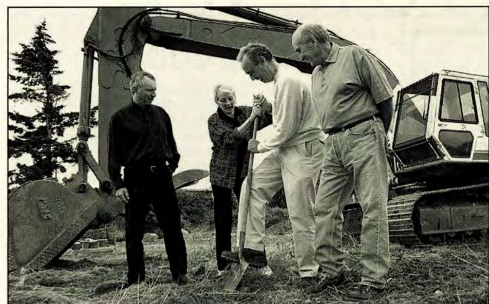
GROUND BREAKING: Symbolically turning the sod at the corner of Lower Ganges and Crofton roads marked the beginning of construction of Heritage Place last Saturday. Doing the honours is Paul Beckmann overseen by Winton Derby, both directors of Long Harbour Ventures Ltd., owners of the project, and business manager Greg Durward. Giving a hand is rental agent Donna Regen of Island Quest Realty Ltd. Photo by Derrick Lundy
