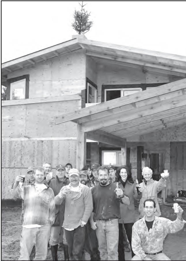
HIGH POINT: Owners, contractors and the architect for the Heritage Place project mark the completion of the highest point of the first of five houses by mounting a tree atop the roof. Heritage Place, located at Lower Ganges and Crofton roads, is being constructed in three phases and when completed will house 45 seniors residents in five separate and independent houses. Balsam House, the first house, will be ready for occupancy in April. Photo by Ellen Young
