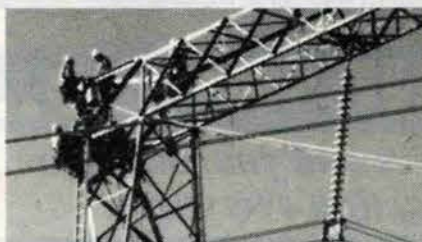
500 KV line repair near Whistler.
