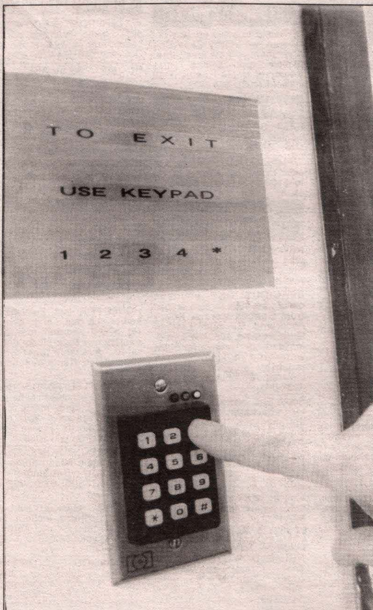
SECURE AND EASY: That's the new keypad exit system at Greenwoods. Residents have to be able to understand and follow the simple directions which are placed next to the keypad, shown here.
