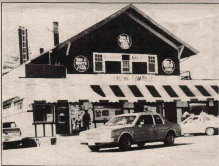
BEFORE THE RENOVATION: The Trading Company building in a photo taken two years ago, when it still sold groceries.
