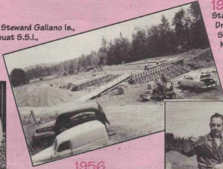
1956 New hospital underway.
