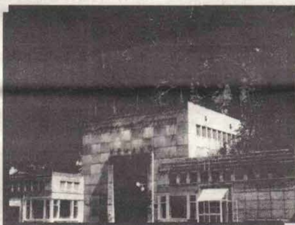
The existing powerhouse is built inside Mt. Dubose; only the entrance is visible outside the mountain.
