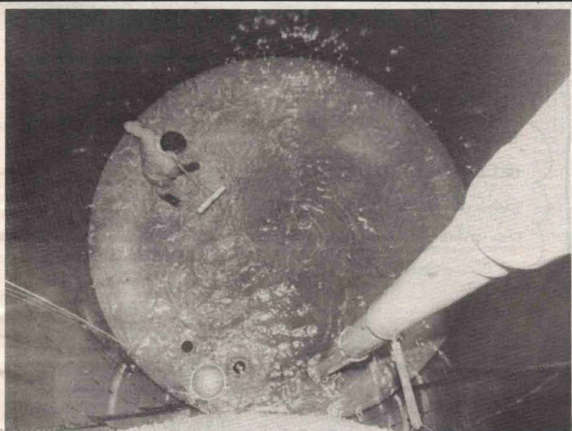
CLEAN WATER: Jack Andrews of North Salt Spring Waterworks scrubs out a 40,000-gallon storage tank on Ganges Hill last Wednesday. Tank cleaning was part of annual district maintenance, which includes flushing water mains. Photo by Tony Richards
