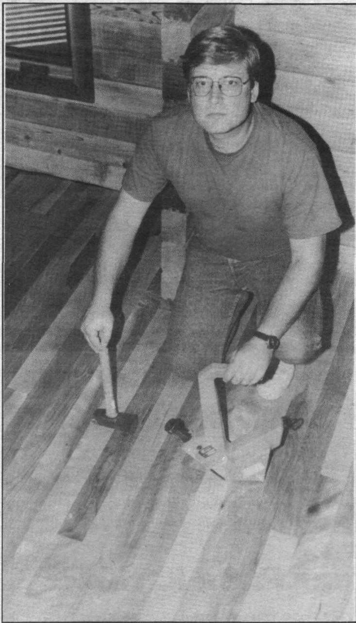
Steve Davison with Mirage floor and tools
