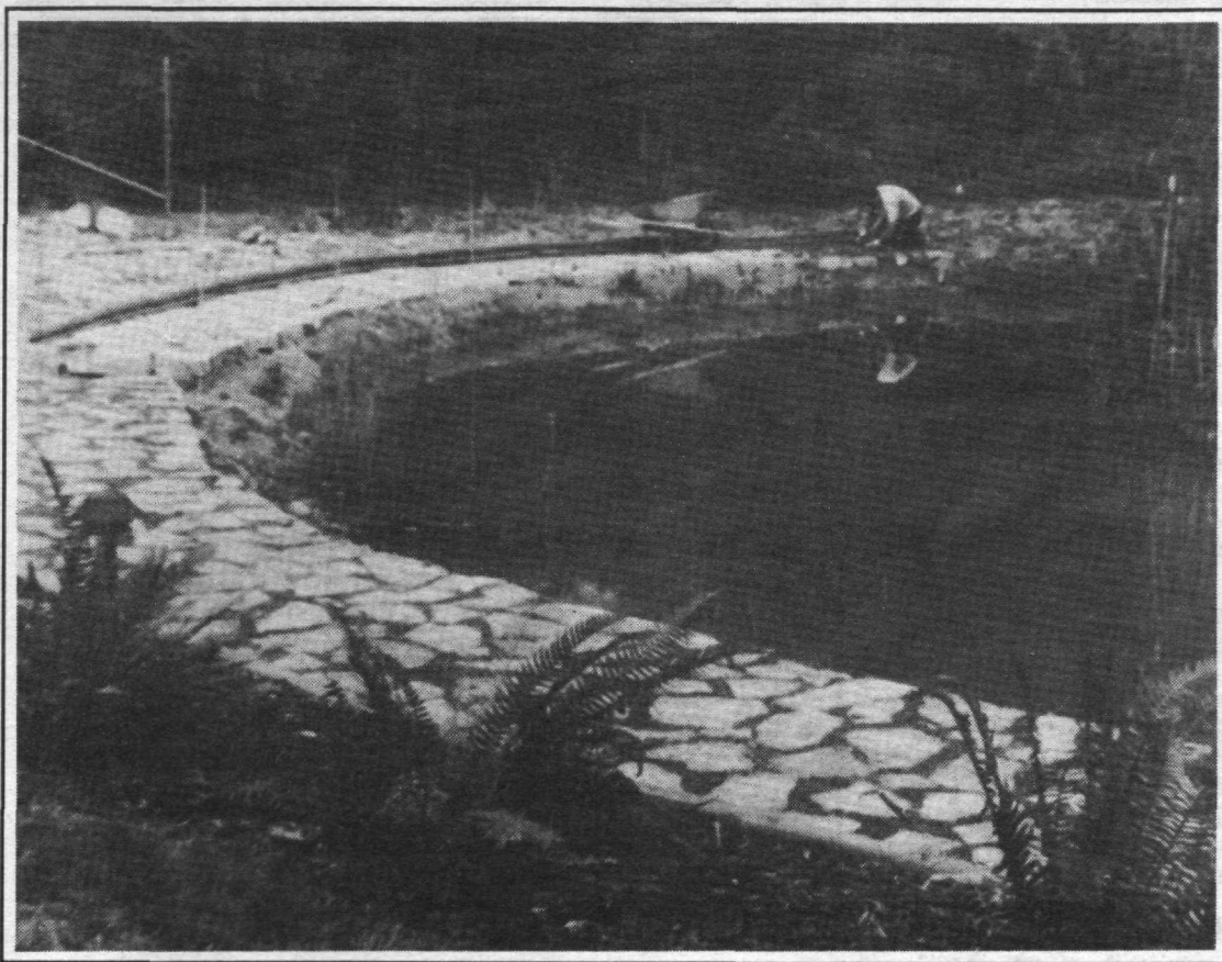
FOCAL POINT: Large pond is the focal point in the back yard of Chuck and Elaine Bell's home. A rock wall is being built around the pond.
