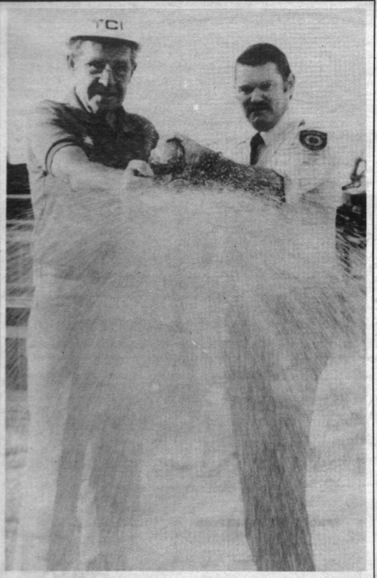
SOD-SOAKING: A ceremonial drenching of the soil Thursday replaced the usual sod-turning as construction started on the new fire hall at Central. Manning the hose are Ben Martens, left, chairman of the board of trustees for the fire department, and Les Wagg, fire chief. The two-day, $180,000 hall is to be completed by the end of November and will complement existing halls at Fulford and Ganges. Photo by Valorie Lennox
