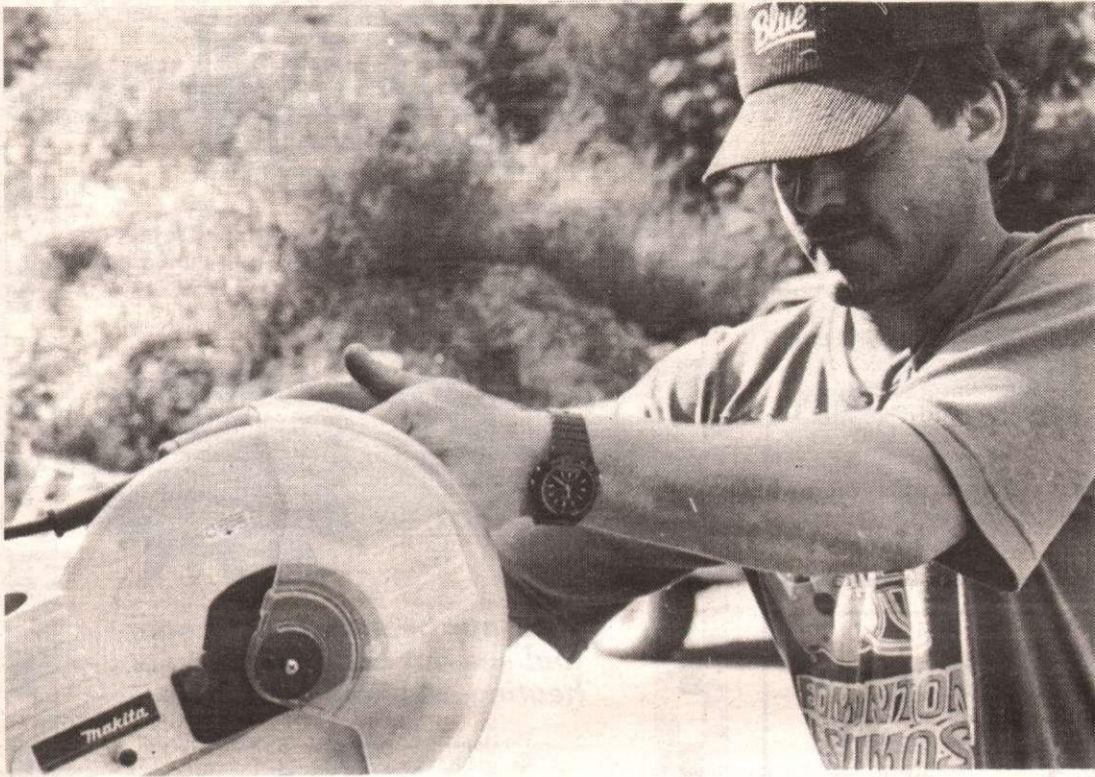
CUTTING EDGE: Barry Byron uses a cross-cut saw to complete trim on a Ganges-area home. Driftwood photo by Derrick Lundy
