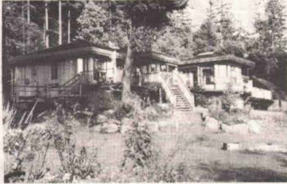
Proposed 20 acre parcel with executive main 2500 sq. ft. main residence and guest cottage.
