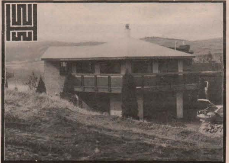
SMITH RESIDENCE, VERNON, B.C.
