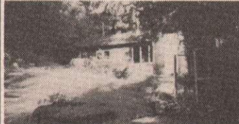
Log cabin with ocean glimpses situated on a high well-treed lot in a quiet area. Part basement. Carport and drilled well. Close to marina and beach. $38,000.
