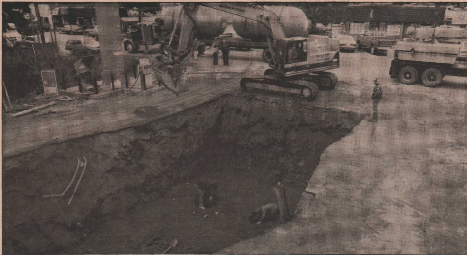
Installation of new tanks at Petro-Canada took place last week.
