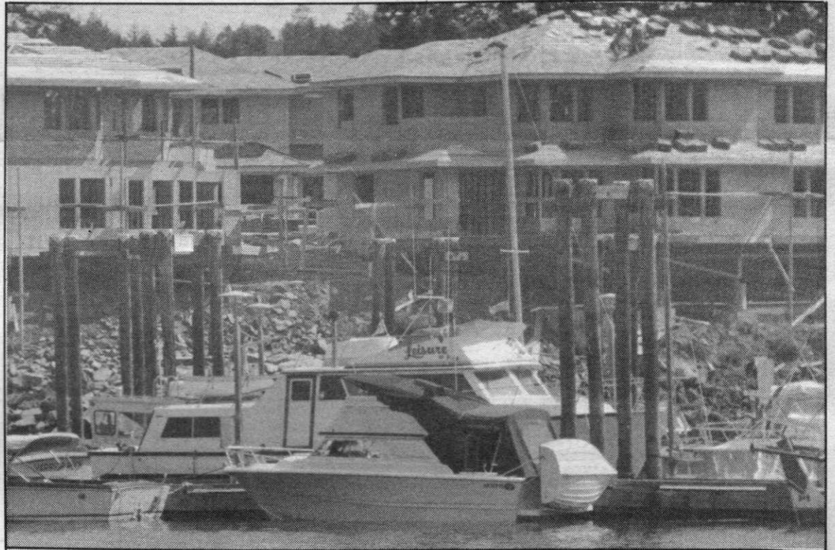
Work continues on Grace Point townhouses in Ganges
