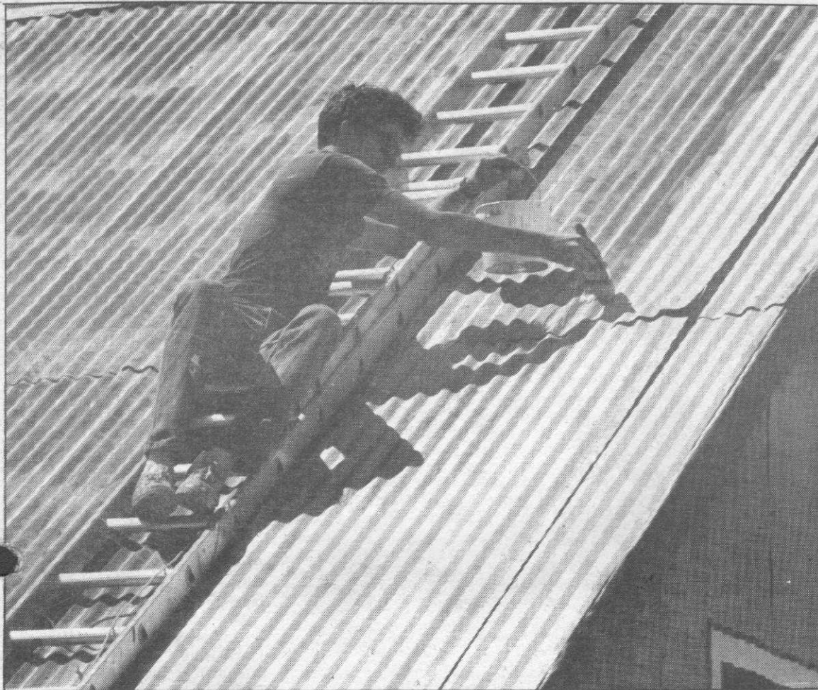
Hot tin roof
