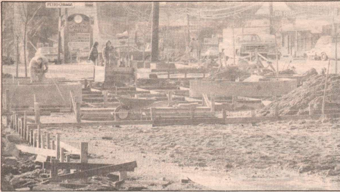
Work at Centennial Park quickly taking shape
