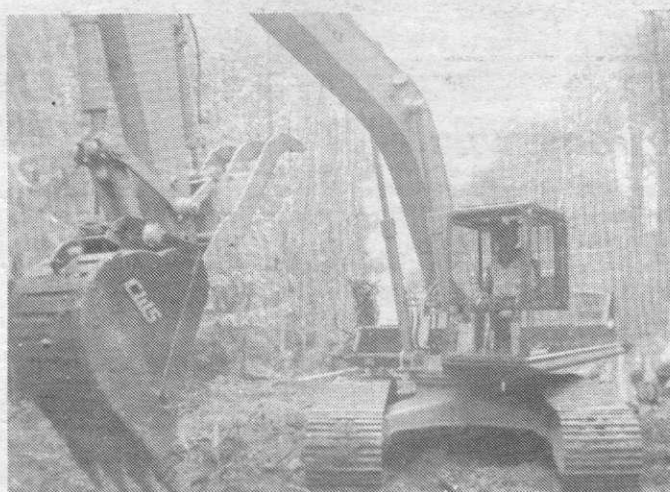
New Komatsu 1-yd. Excavator with Hydraulic Thumb
