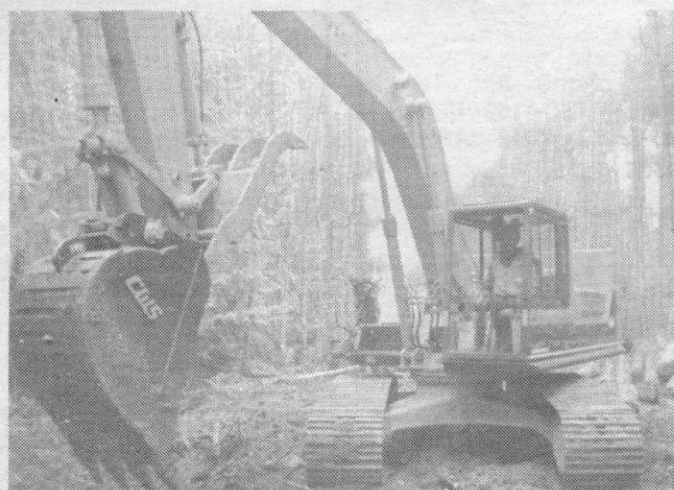
New Komatsu 1-yd. Excavator with Hydraulic Thumb
