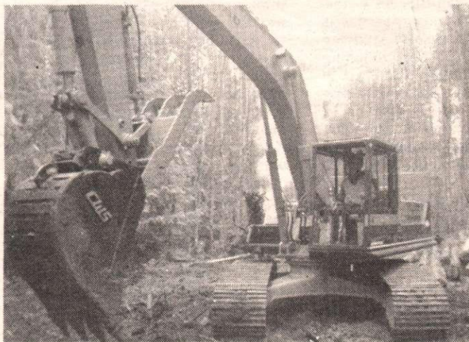
New Komatsu 1-yd. Excavator with Hydraulic Thumb
