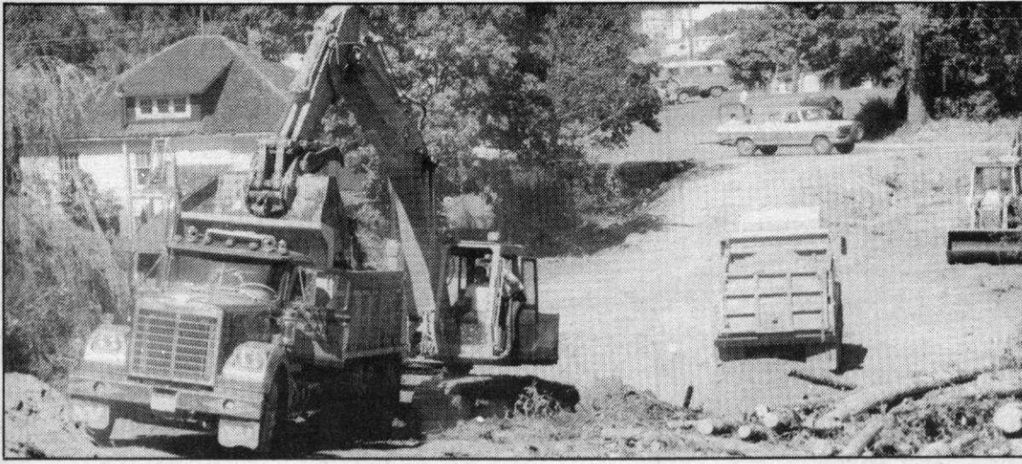
Work under way on extension
