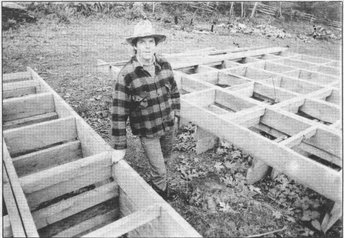
Chris Hatfield with wooden pens being constructed at Yeo Point salmon farm
