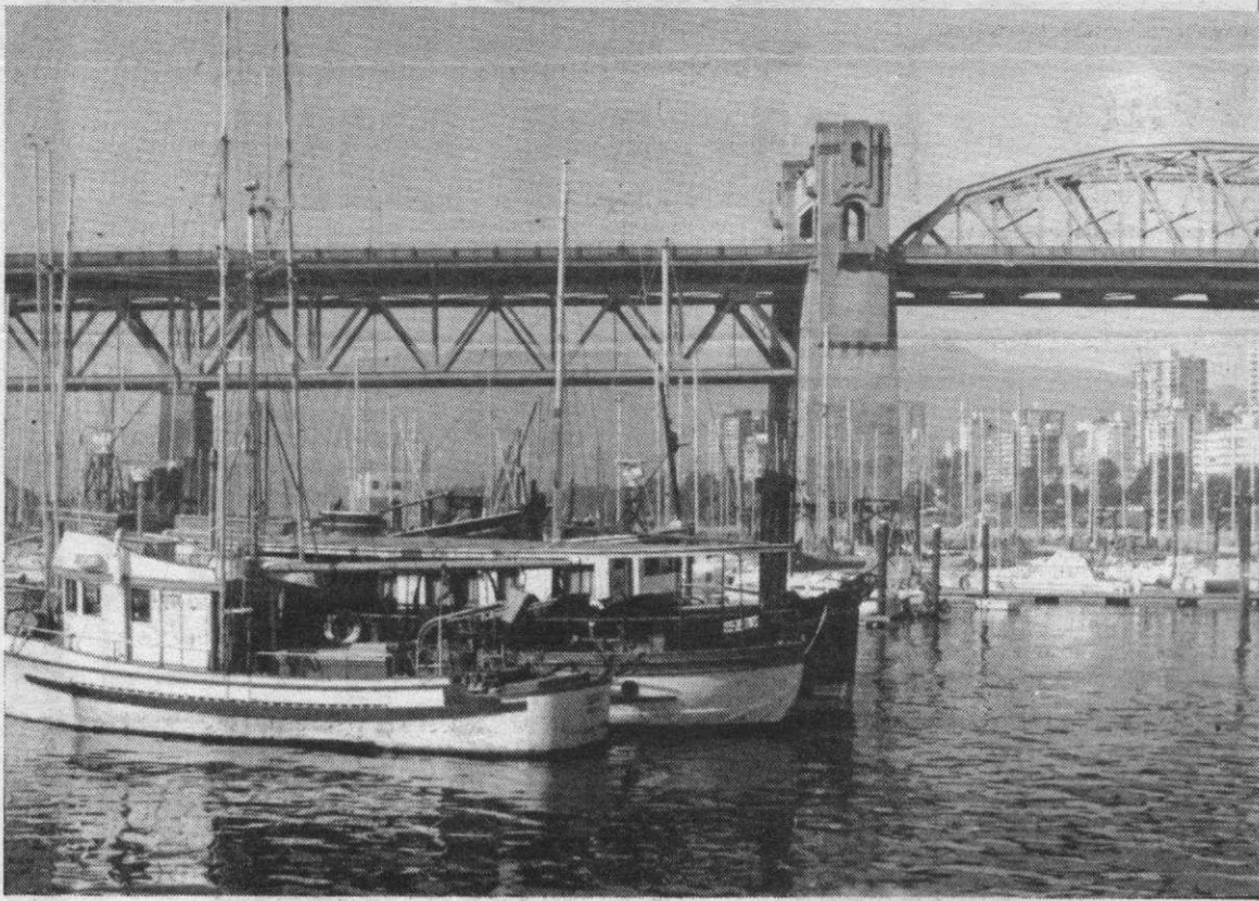
When the project is completed and under way, the marine facilities in False Creek will enjoy the closest view of the installation. This is the other side of the water.
