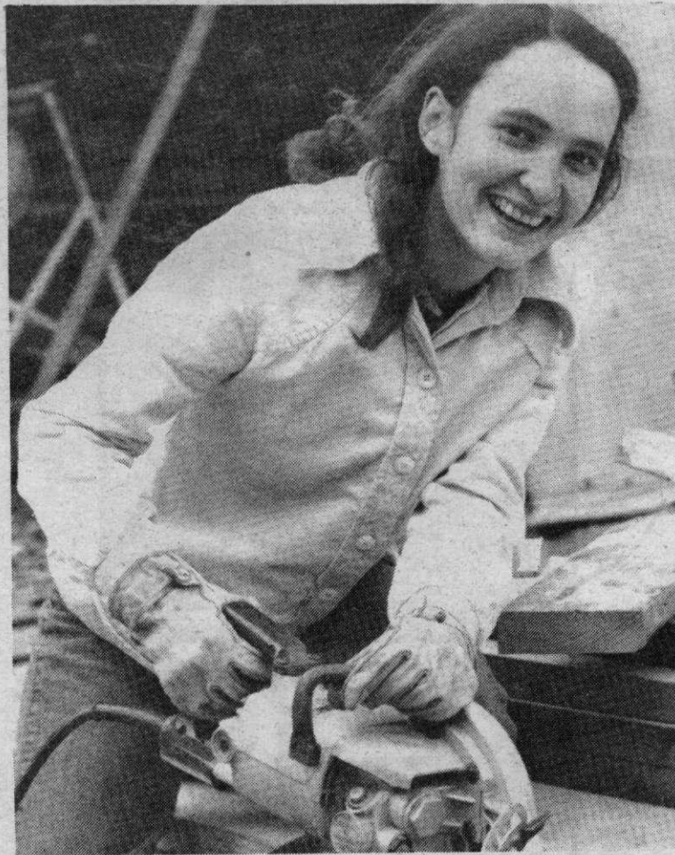
Above, crew lays the first board of the sub-floor. Nicholas Gaitt, standing, and Diane English, sitting in front, are joined by Bob Andrew, Corky and Lisa Hughes. In photo below, Diane wields a power saw to cut stakes.
