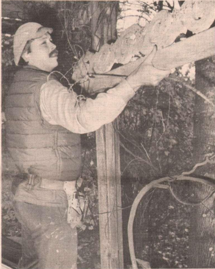
Art Lucs removes original gingerboard from front porch.
