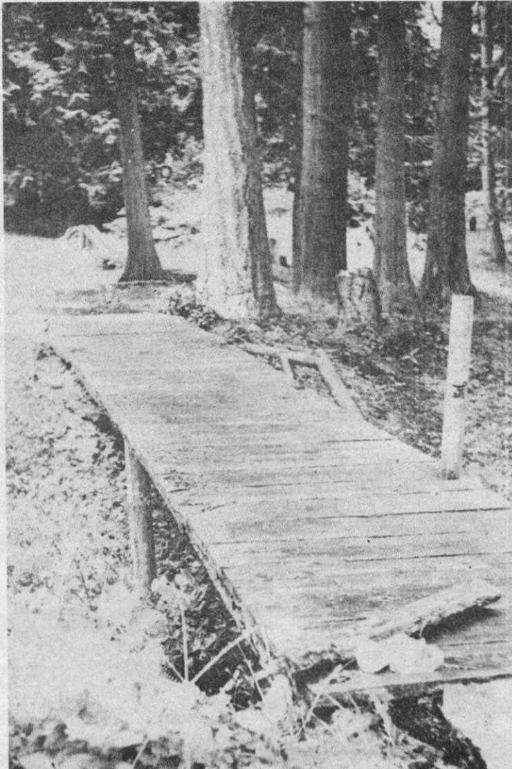
Vandalized footbridge in Centennial Park on Galiano Island.
