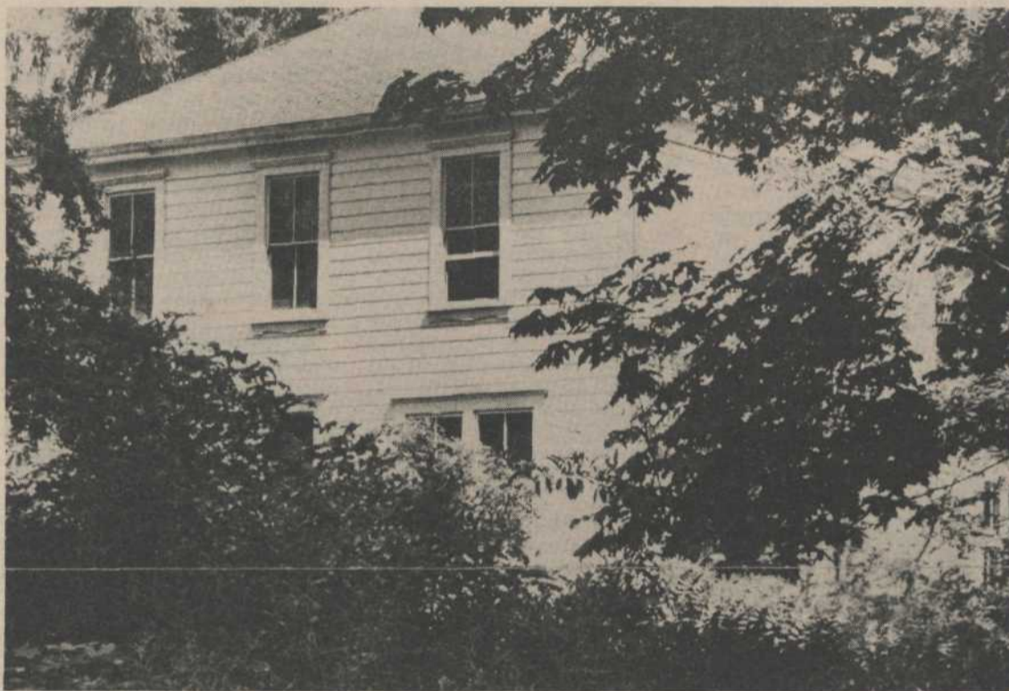
Half hidden by trees is home of Guy and Margaret Cunningham, former Stevens Boarding House.
