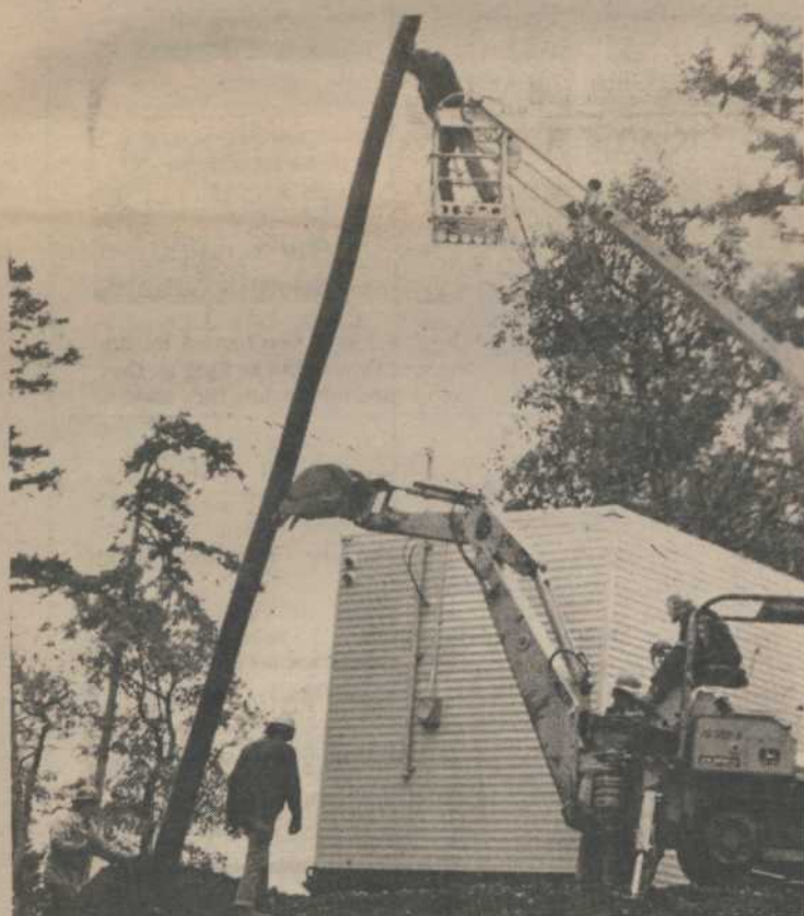
Pole goes up at Galiano for new telephone line
