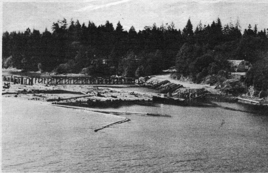
Logging installation at Welbury Bay has been the subject of heated protest by residents of the bay. The
