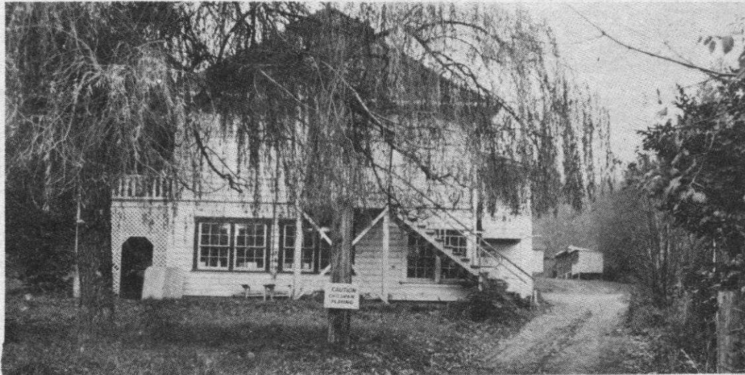
Salt Spring Island Community Centre on Ganges Hill.
