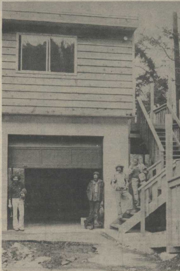
Health Centre is almost completed at Saturna Island. Erected above the island's fire hall, the new facilities have been partially paid for out of a Canada Works grant.
